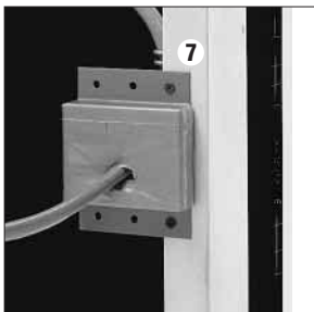
The bracket mounts directly onto the stud.
