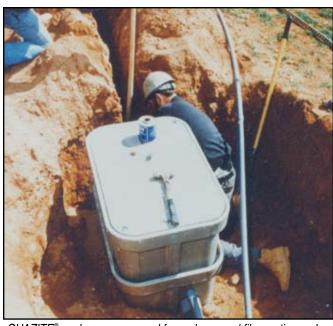
QUAZITE® enclosures are used for underground fiber optics and electric cable.
