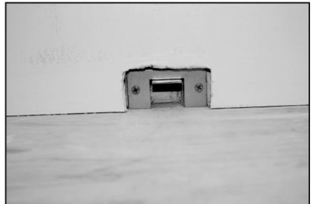
Install Nail Plate
