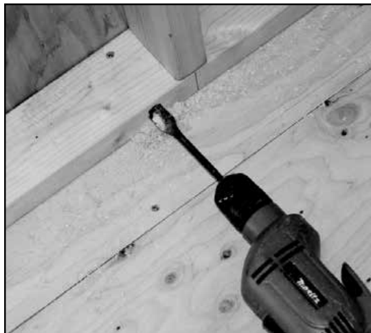
Drill Horizontal Hole
