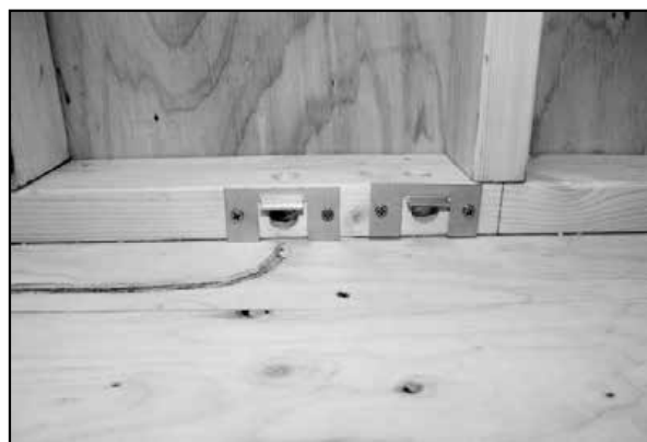
Install Nail Plate
