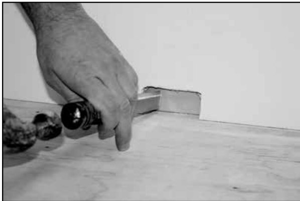
Chisel channel
