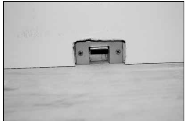
Install Nail Plate
