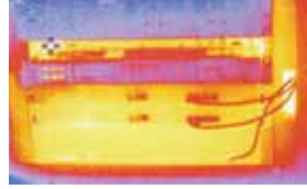
Data Center Thermal Mapping
