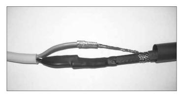
4. Shorten (cut) the ground braid strap on the heating cable so that ground braid strap and ground lead butt at the splice centerline. Tightly twist the ground braid strap. Crimp the ground braid strap to the ground lead using an un-insulated splice connector. Secure connector at the indented area with one and a half wraps of fiberglass tape (not included in kit).
