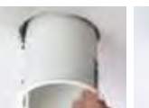
Insert housing into position and align slots in housing wall with indicator label on inside of plaster frame opening (bottom of cam lock spring blades should be positioned on flat area of the plaster frame). Then secure in position with cam locks.
