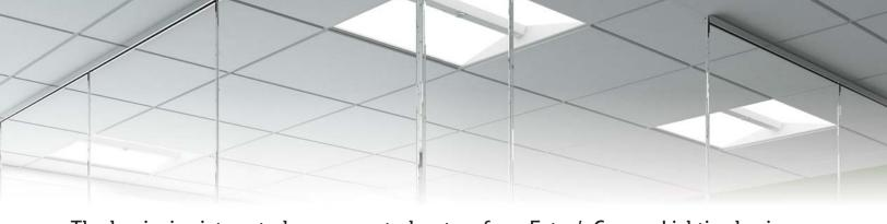
The luminaire-integrated sensor control system from Eaton's Cooper Lighting business reduces the design time and complexity of meeting energy codes for both lighting and controls. The sensor system was designed to guarantee occupancy and daylight harvesting coverage from within the footprint of Metalux ambient luminaires, so the lighting design is the control design. And, the system achieves the lowest installed cost in small spaces compared to traditional control products.
