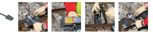
• Used to remove the slag from the crucible area of the mold after making a ERICO CADWELD connection
