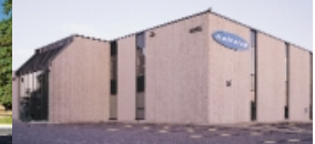
Banner Manufacturing Plant Minneapolis, MN
