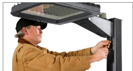
Tighten bottom bolts and complete wiring.
