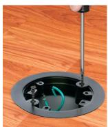
4 ...with the two #8 x 2-1/2" screws provided. For textured or grooved flooring use caulk as required under the leveling ring.
