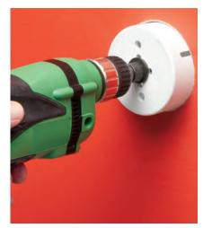
Determine bracket position. Cut opening with a 3.5" hole saw.
