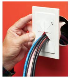
...through the slotted opening in CE1RP. Insert into hole. Level, straighten the bracket.
