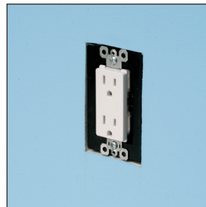
After drywall installation is complete install receptacle and cover.
