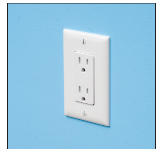
After drywall installation is complete install receptacle and cover.
